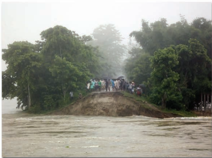
Dhemaji- Brahmaputra River's embankment breached
